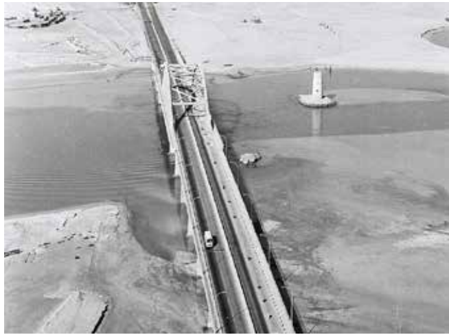
Al Maqta Bridge, built in 1967, was the first connection between Abu Dhabi and the rest of the Emirates, bridging seas and eras.
